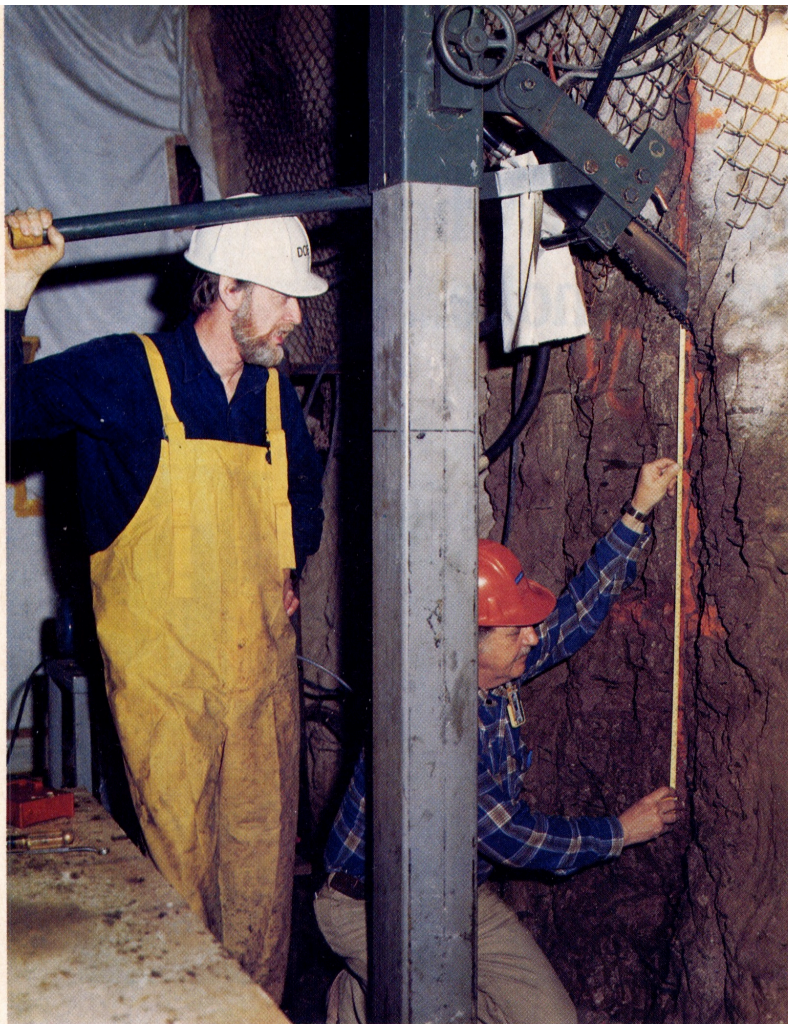
With a diamond-tipped chain saw (embedded in the rock wall at upper right), technicians are able to cut large blocks of rock for testing.
